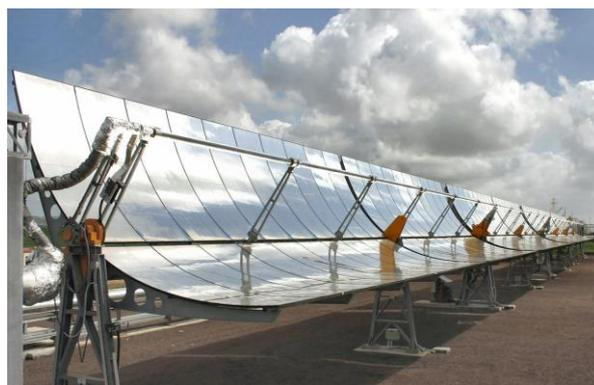
Fig.1 – CSP Parabolic Trough Solar Collectors
