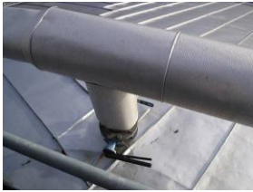
Collection over digester
