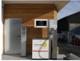
Biogas service station
