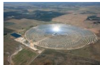
Gemasolar plant. Power tower
