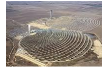
PS20. Power tower
